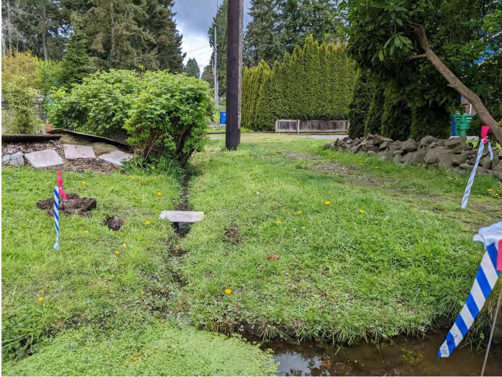
Photo 3. Dredged swale connects to Ditch 1, photo oriented west.
